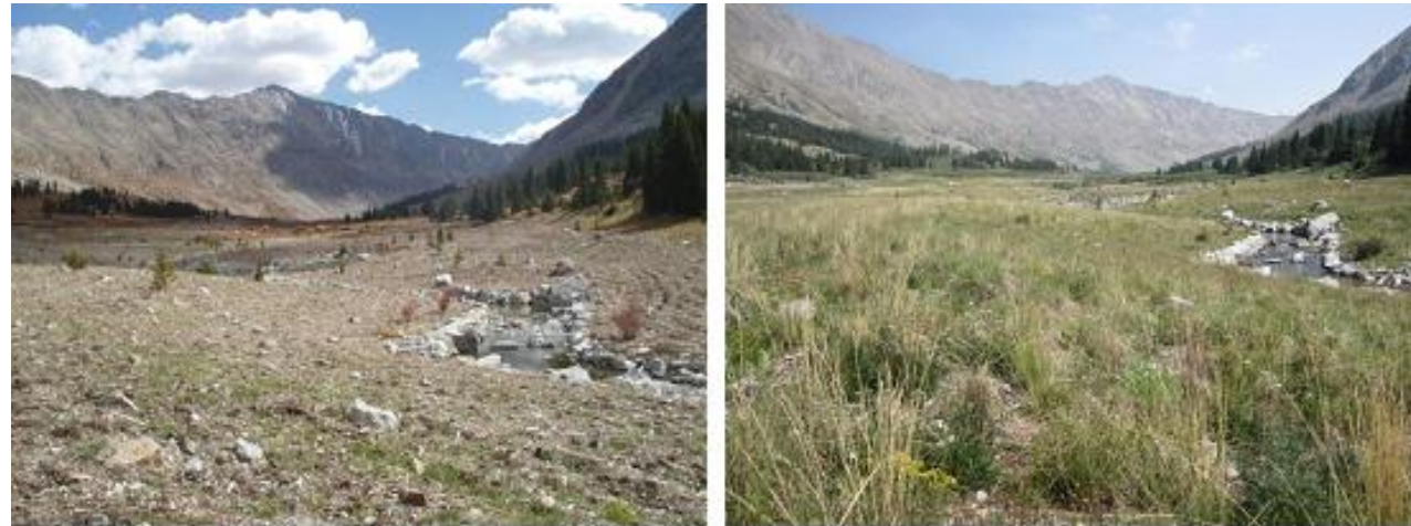
Storke Yard at Climax in 2008 (left) and in 2012 after revegetation activities that included using compost produced at the site's award-winning Biosolids Composting Operation. These activities were part of a larger project to restore the Arkansas River channel and habitat at Storke Yard, both of which had been impacted by historic mining activities.
